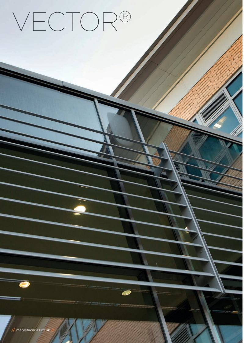
Vector® is a versatile brise soleil system featuring aerofoil or rectangular profiles and is suitable for all building types.
