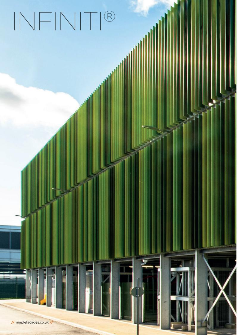
Infiniti® is a continuous, hidden-fix brise soleil solution for all building types, particularly occupied public buildings. The system offers a wide range of design possibilities for vertical or horizontal layouts, with minimal fixings to help meet budget requirements.
